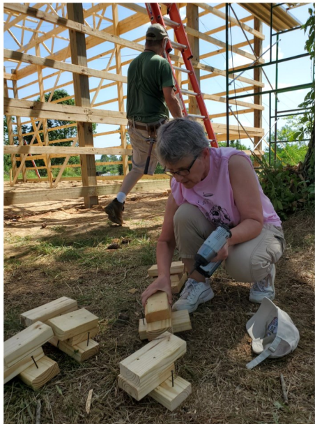
Sr. Cathy Bauer rebuilding a barn in Mayfield, KY
